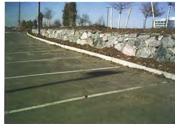
EXAMPLE OF STONE RETAINING WALL.
