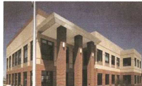
EXAMPLE OF TWO-STORY WITH BRICK ENTRY AND BRICK ON LOWER LEVEL
