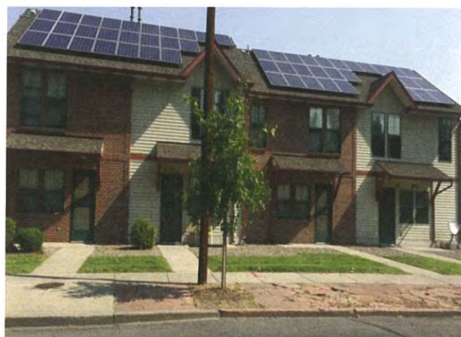
EXAMPLE OF TOWNHOMES WITH SOLAR
