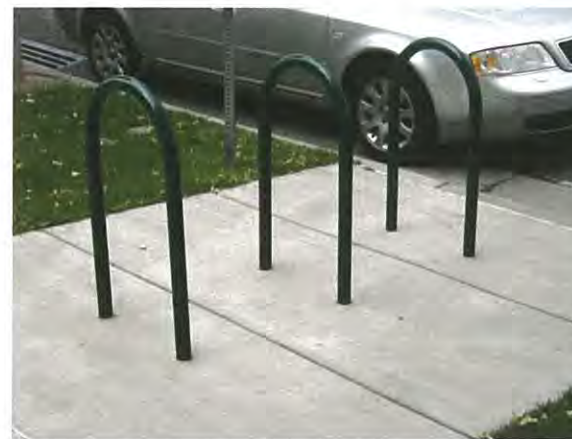
INVERTED 'U' STYLE BIKE RACK USED FOR VARIOUS BIKE TYPES AND SIZES.
