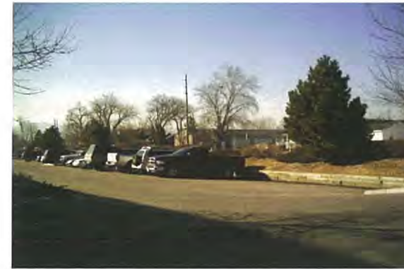
PAVING AREAS LOWER THAN PERIPHERAL ROADWAYS.
